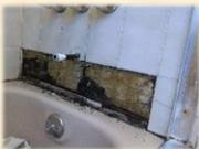
But if the seal around the bath or shower tray is old you won't see the effect of it (though you'll probably smell it). A leaking pipe behind the bath or under the sink can be hard to spot too.
